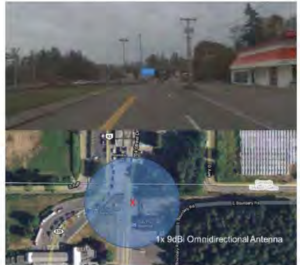
Figure 4-6: SR 539 U.S.-Canada border Bluetooth installation location
